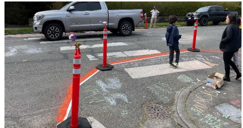
A low-cost ($250), short-term set of bump outs installed by concerned neighbors in Anchorage, AK.
