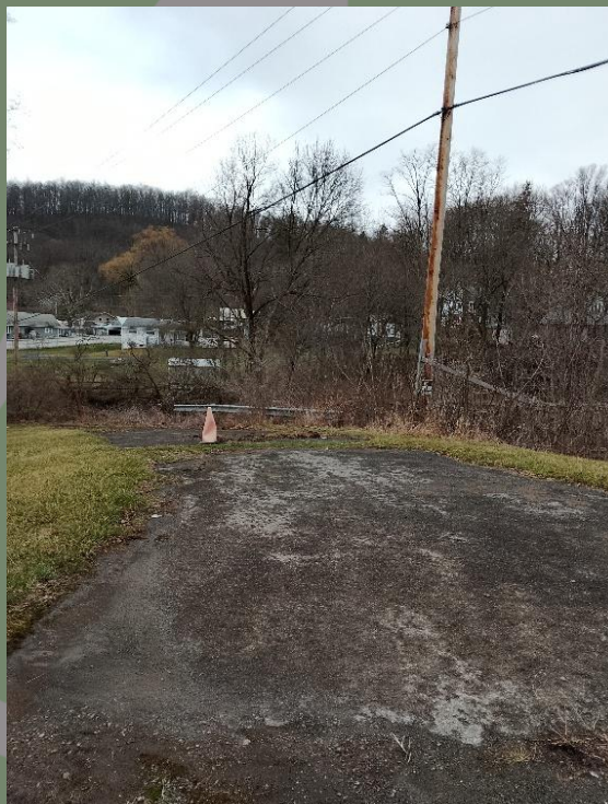
Area in front of the old pedestrian bridge, looking across to MacDowell Road from Main Street
