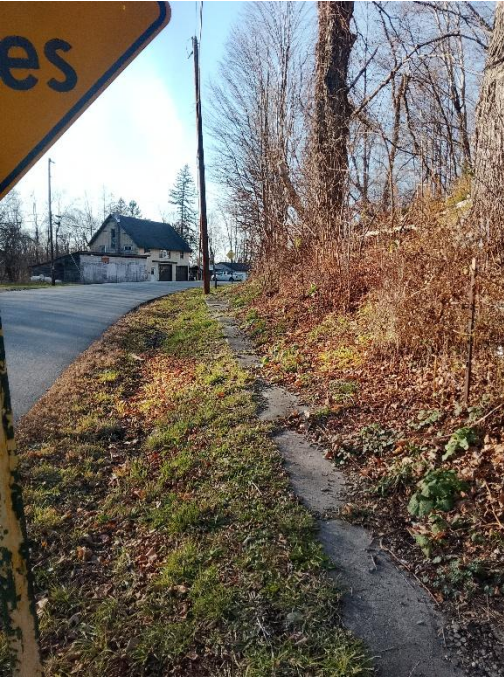
A thin, overgrown sidewalk along Brooklyn Terrace to a barely-there staircase leading to a now vacant lot
