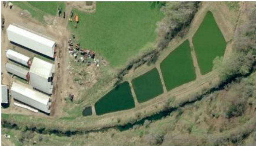
The wetland was separated into five segments to allow retardation of water flow, which prolongs biological activity and enables sedimentation to improve water quality.
