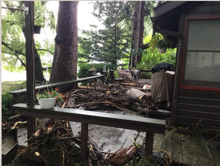
August 2018 (Source: Mecklenburg Fire Department)
