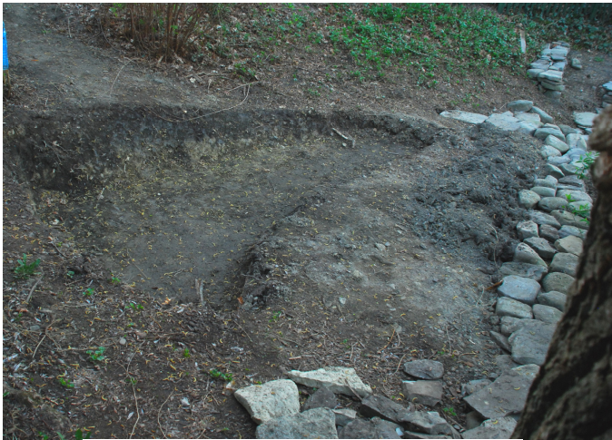
The rain garden is dug and bermed.
