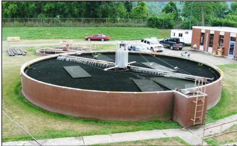
Trickling filter for Village of Addison Wastewater Treatment Plant; ring levee (by the fence) provides flood protection (courtesy of Village of Addison).
