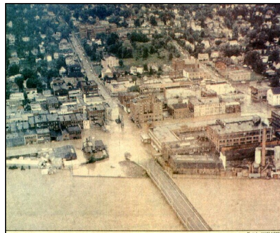
View of the Market Street area of Corning, around what is now the Centerway Square, when the Chemung River overtopped the levee in 1972.
