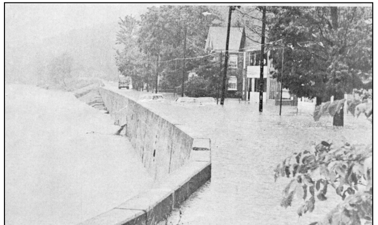
During the Agnes flood, the floodwall kept the Canisteo River out of Hornell, but trapped runoff from the surrounding hills.
