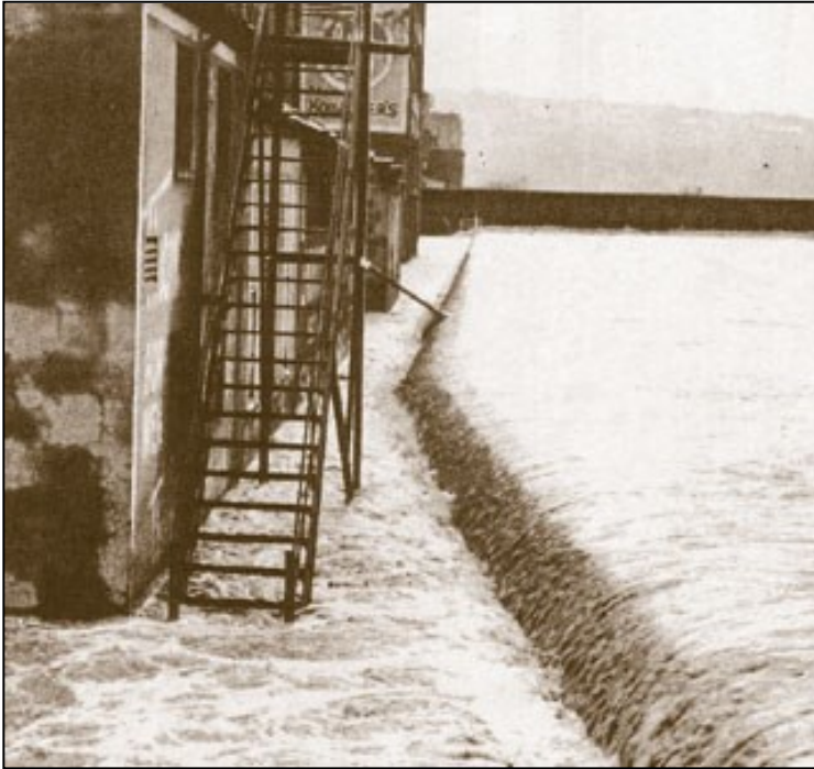
The 1972 Tropical Storm Agnes flood overtopped the floodwall in Elmira.
